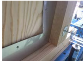
(c) 鋼製枠の座屈
